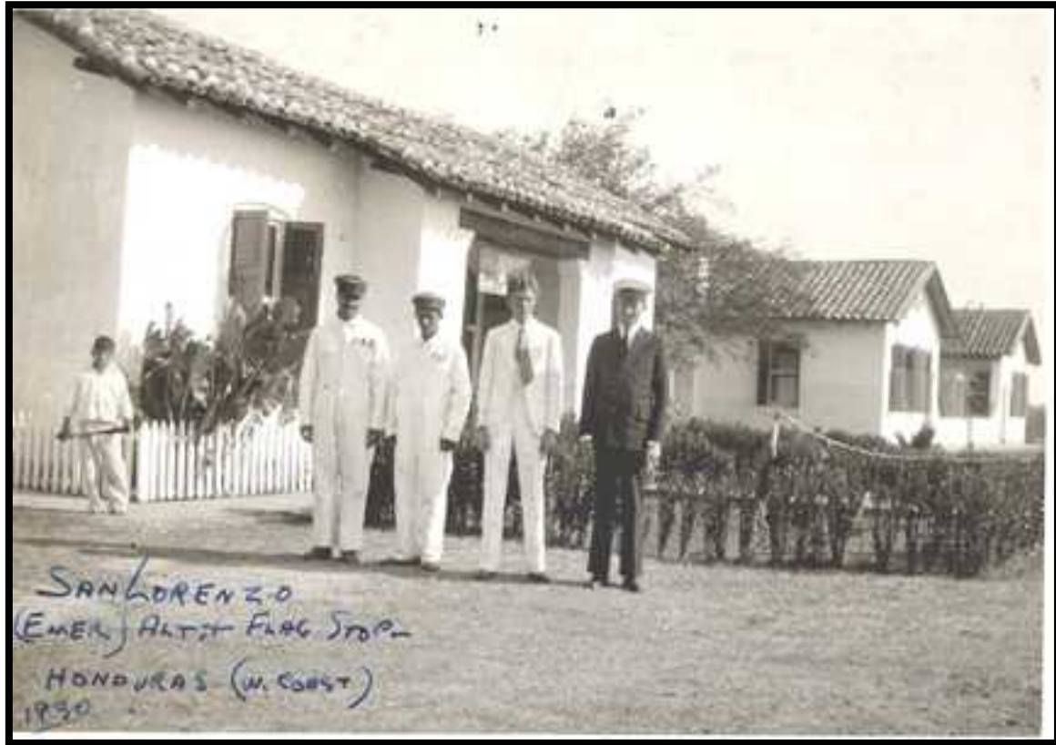
Fig. 3. PAA installations in San Lorenzo.
